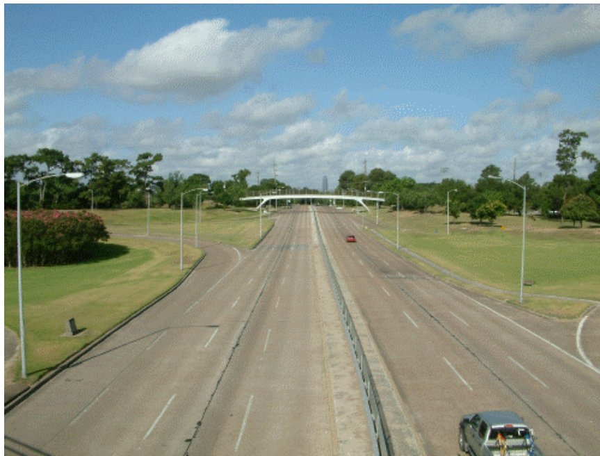
Photo 1.2 – Memorial Drive, limited access parkway
